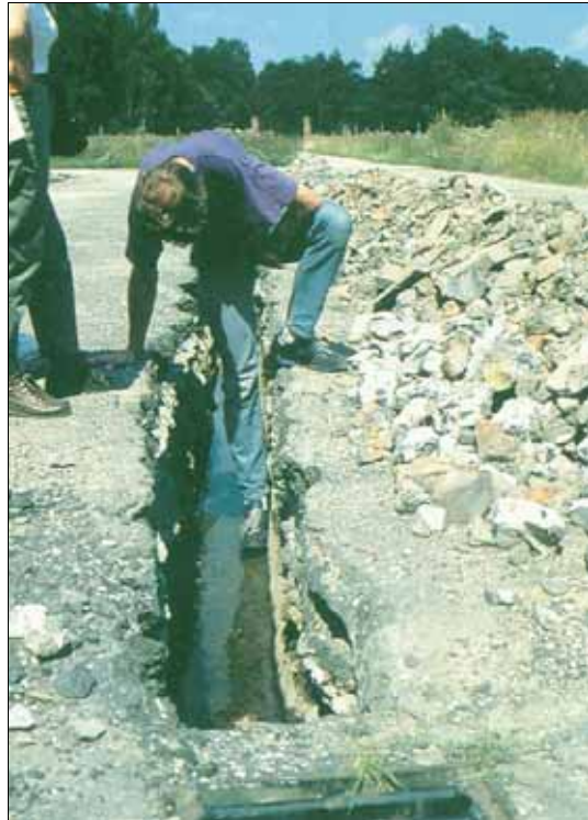
Fig. 57: Then and today – the unchanged ground water state in the Birkenau camp, here in midsummer 1991, in a construction trench in front of the Zentralsauna, approximately 70 cm. Incinerations of corpses in pits many meters deep, in accordance with witness testimony, were not possible.
