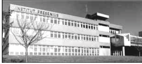
The masonry samples taken by Rudolf were analyzed by the renowned Institut Fresenius.
