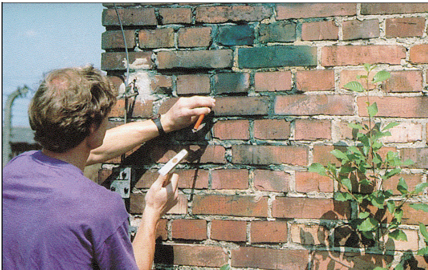
Fig. 68: The outside of the external wall of hydrogen cyanide delousing wing of building 5a in August 1991. Small amounts of cyanide which diffused through the walls are discoloring them at places still today. 50 years of the most detrimental environmental influences did not change this fact.
